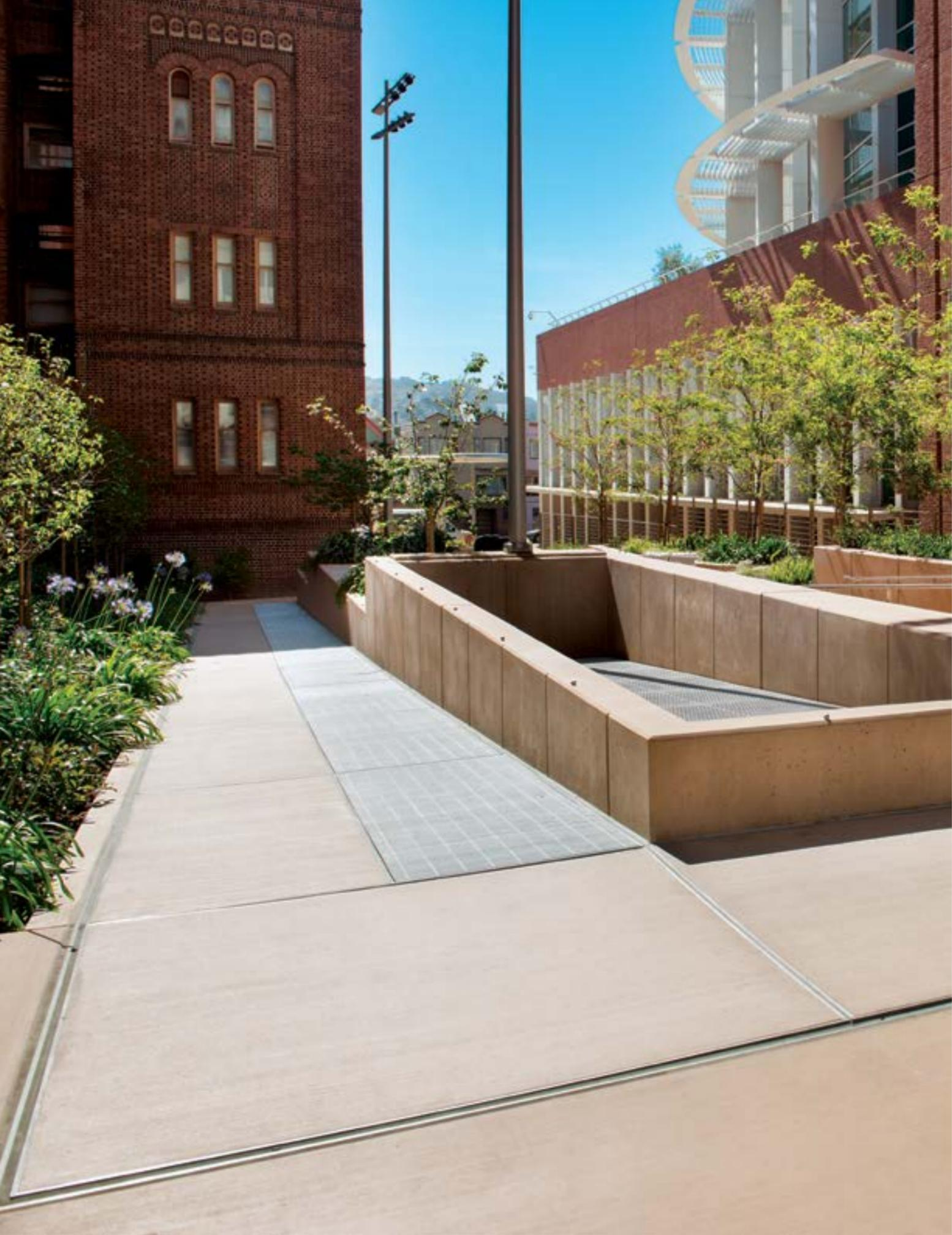
One of the largest base isolated hospitals constructed in the United States—able to glide 30 inches in every direction during a seismic event
